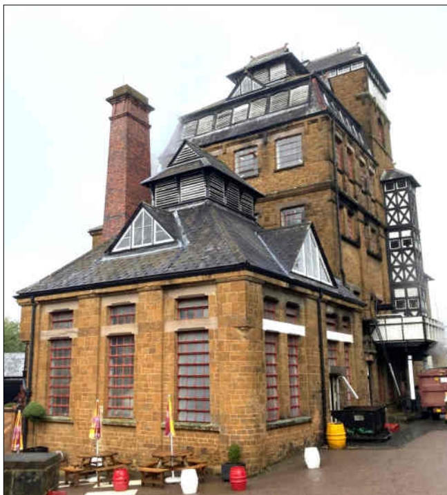
The tower brewery is characterised by a multi-storey design that uses gravity to aid the brewing process. (Photo by Pete Flynn)
