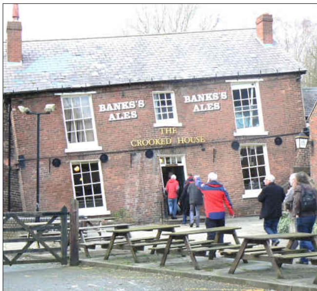
The Crooked House near Dudley in the West Midlands before it was illegally demolished in August 2023.
